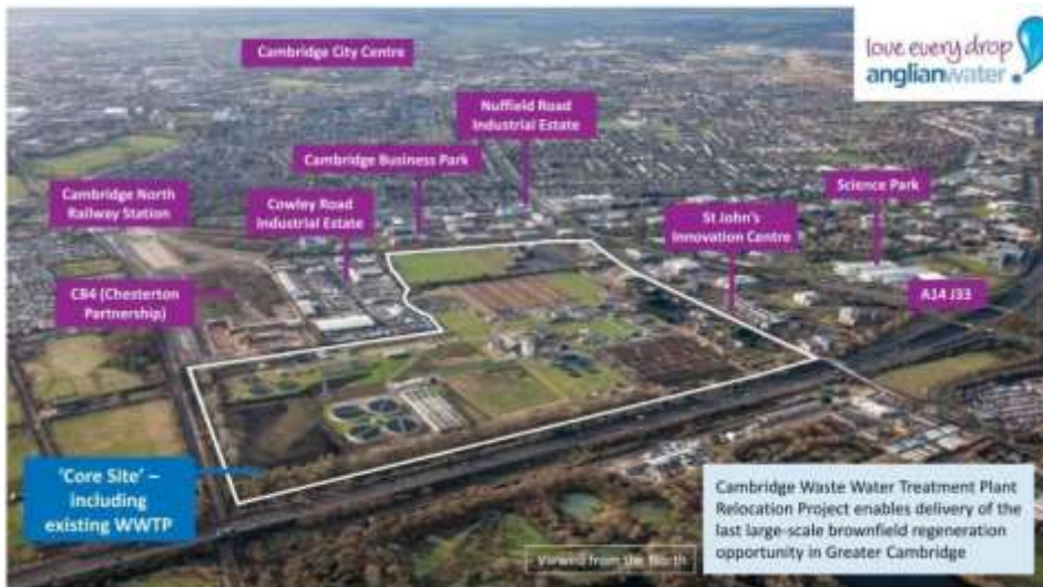
Figure 2: Detailed aerial view of existing Cambridge site .
